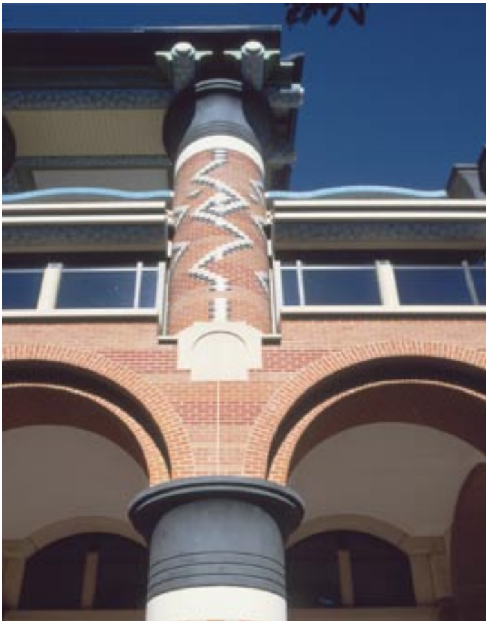
The Tumbling Stream and Confluence fall to the Lazy River over the Balcony of Appearances of Meeting Room 1.
