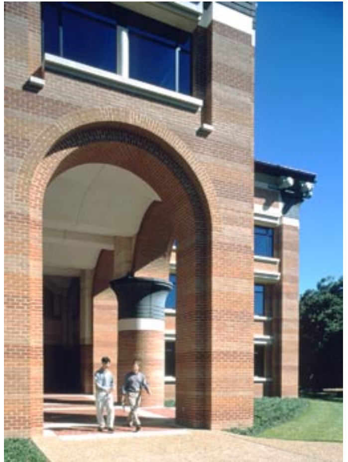
The other extremity of the 300'0" (100M) - long Arcade faces West - towards the main body of the Campus buildings. The Arcade vaulting is plastered so as to look 'internal', and therefore welcoming. It also gives a white surface for the decoration that will come when its conceptual function is appreciated and understood. The curving edge of the 'ground-cover' discs can be seen.
