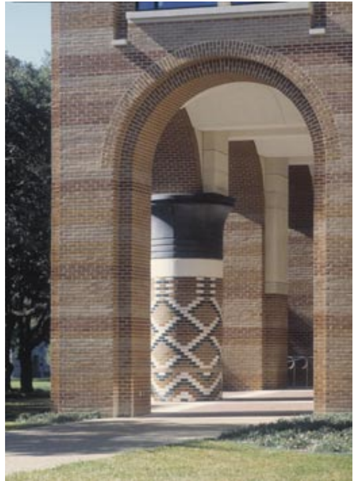
The double-height Arcade of the Southern Portico, in front of the main door, seen from the Eastern side. The 4-colour St. Joe's bricks and creasing tiles represent the sedimentary 'Submarine Mountain' which entombed the Genius Loci prior to its release by the Architecture of the Ontogenic narrative at the Time of Inception.
